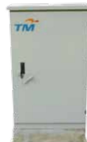
FIBER DISTRIBUTION CABINET (FDC)
